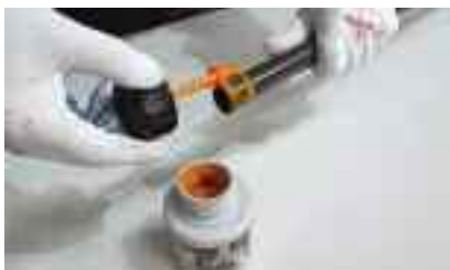
7. Apply solvent cement to fitting and pipe.
