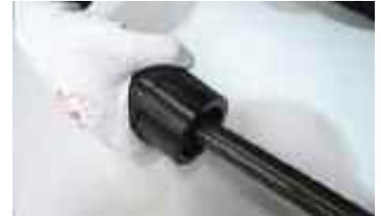
3. Chamfer and trim end of pipe.
