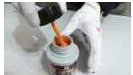
6. Stir solvent cement.
